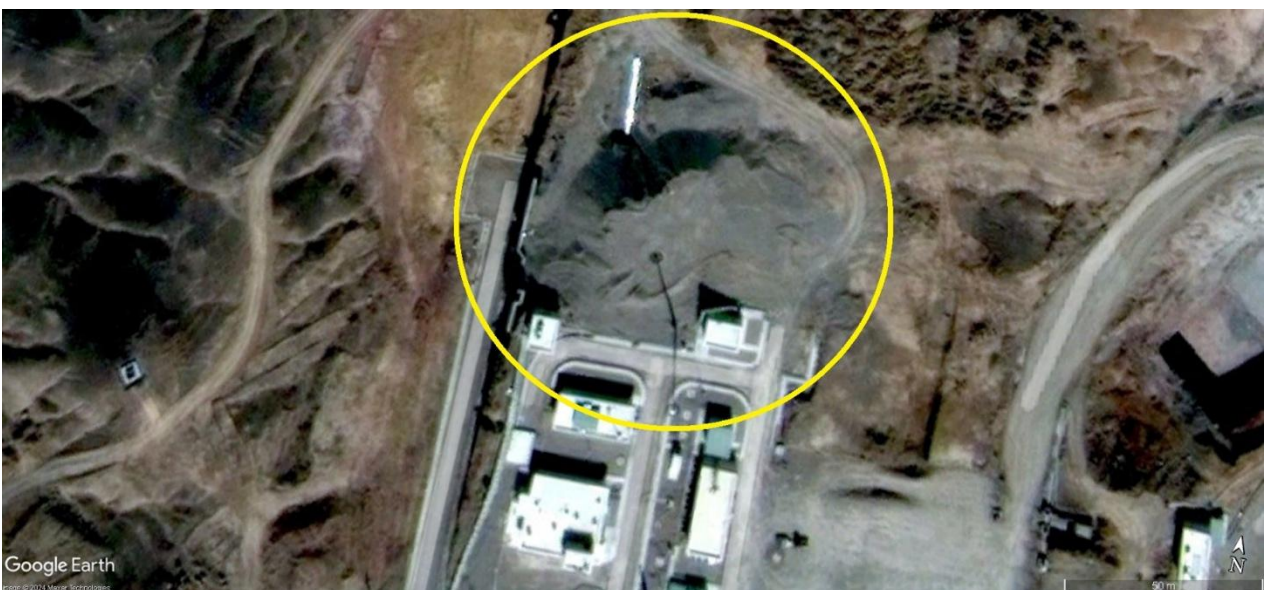
The imagery of the 2012 Semnan site after the underground facility was wholly covered with soil
