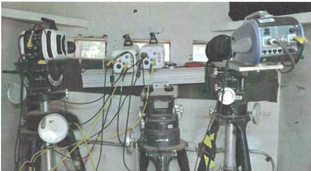
Figure 30: Cameras installed in instrumentation bunker.
