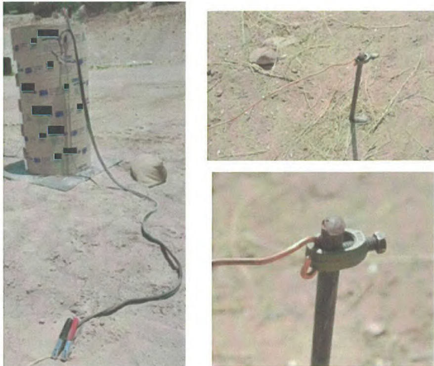
Figure 37: ESD protection (lead is attached to conductive tape, wrist strap and copper wire connected to grounding rod).
